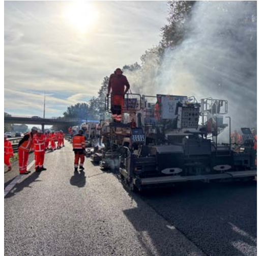
Asphalt Recycling Train (ART)
